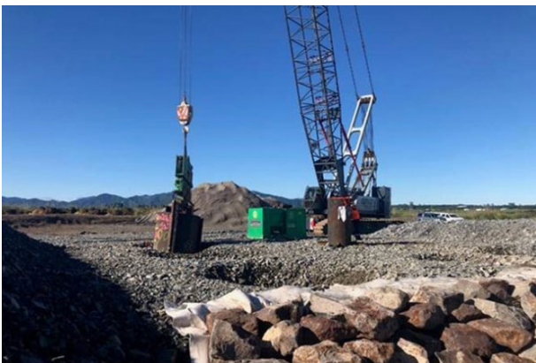
Figure 5: A DC trial was conducted on site to assess the likely depth of improvement and potential damage to geotextiles.
