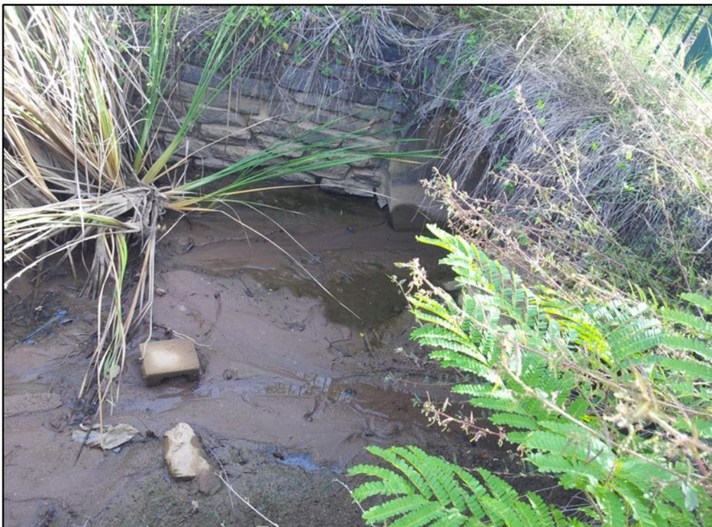
*Inlet Zone at Fairway Waters in Durack Illustrating the High Sediment Loading of Incoming Waters*
